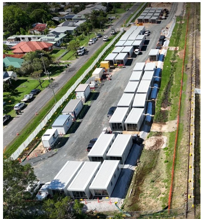
Photos: Aerial images of Prince & Station Street Village
